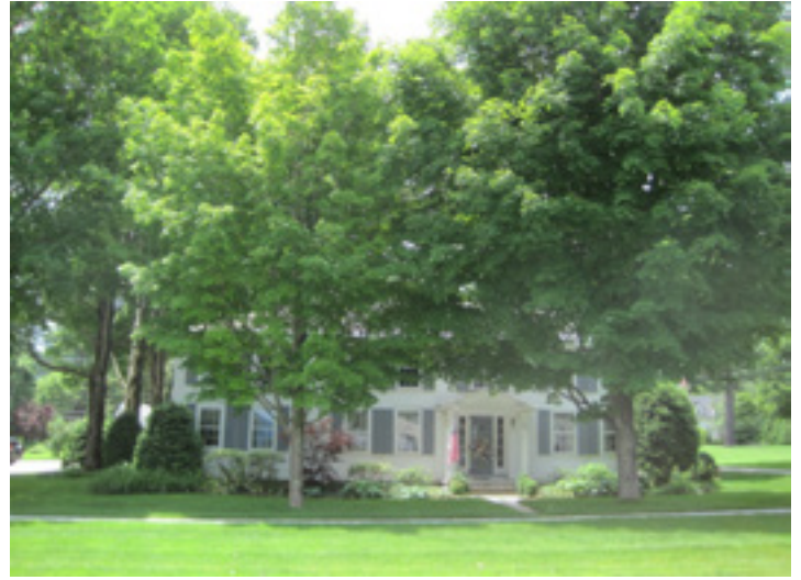
Full Front View: note the screened porch has been removed; also, the door overhang and the trees have dramatically changed from the 1925 picture below.
